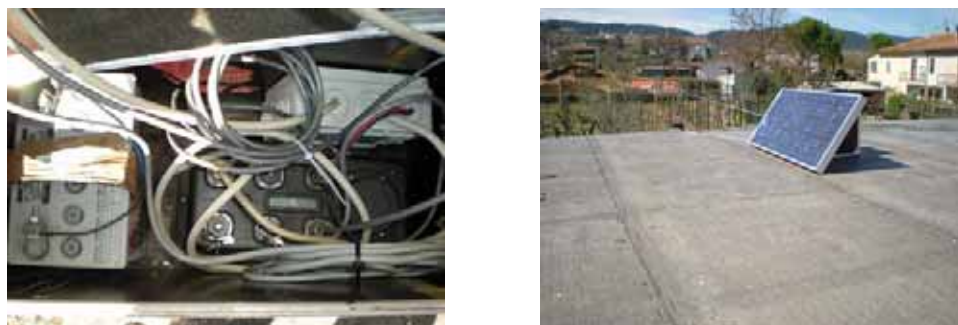
Figure 6.10 Example of installation of NRN3 station equipped with solar panel.
