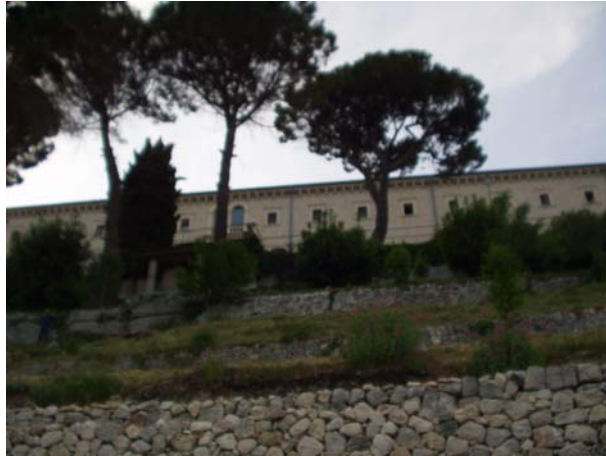
Figure 46. Location of the RAN station, at the edge of the terrace where the Montecassino Abbey is located
