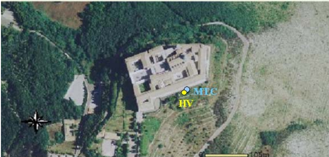
Figure 44. Location of the RAN station and of the corresponding single station ambient vibration measurement
