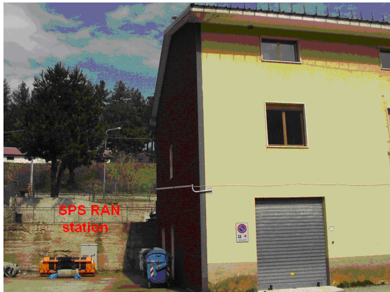
Figure 5. Location of the Spezzano Sila RAN station
